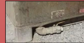
Screw Off Elbow Increases Chance of Leaking
